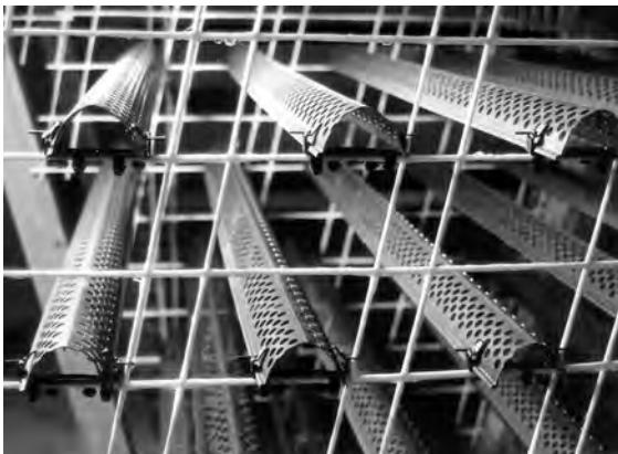
FIGURE 1B Splash fill installed
